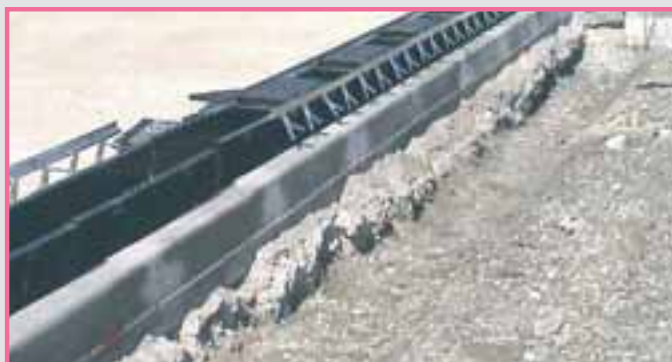
(FIG. 1) • MUFLE DRAIN INSTALLATION UNDERLYING LAYER
